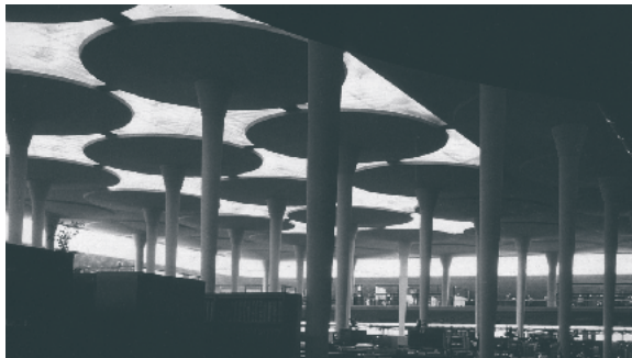
Johnson Wax Building en Racine. Exterior, perspectivas e interior
